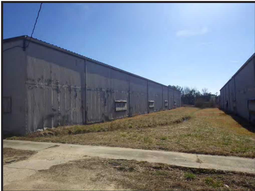
Figure 23. Typical Window Openings, Warehouses 3 and 4, Looking South
