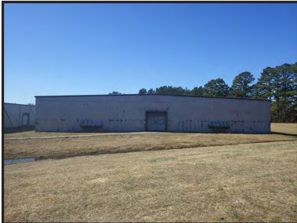
Figure 21. Warehouse 10, East Side
