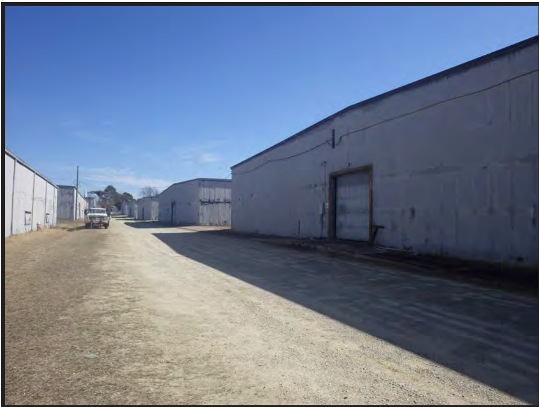
Figure 19. Warehouses 1-6 Looking East
