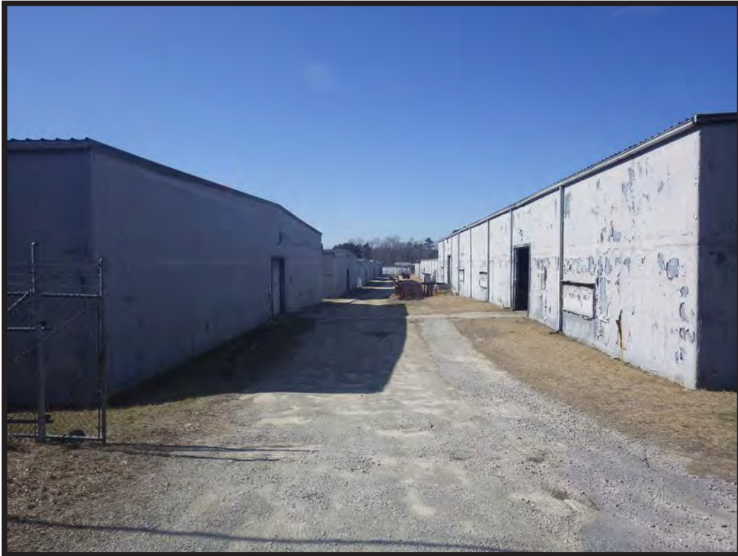
Figure 18. View From Bridge Street Gate Looking West
