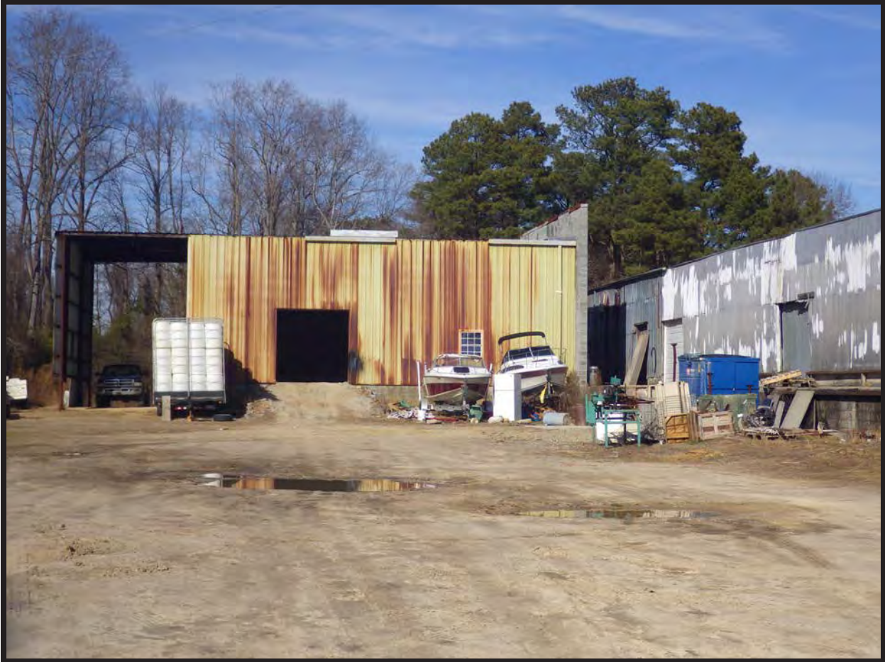
Figure 16. Metal Warehouse, South Side
